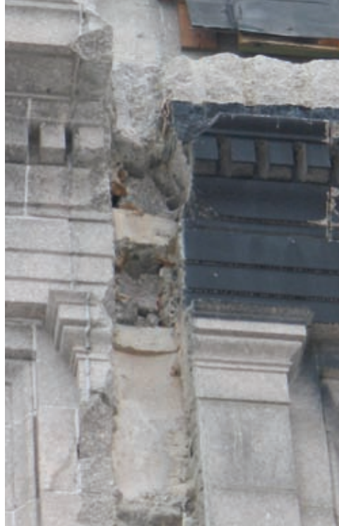
At left, damage to the outside of the building. Right, repairs completed by Phoenix Bay State Construction Co.
